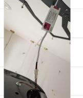
3. Find the largest lampshade, that is, the one with a small hole in the middle, fix the light source and the light source to the lampshade, and then connect the driving wire of the upper ceiling to the following picture, and hang the largest lampshade with the light source box to the ceiling.
