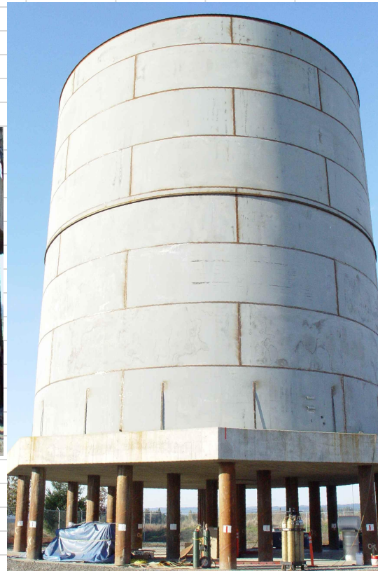
Figure 54-4 Tank Elevation Looking Northwest
