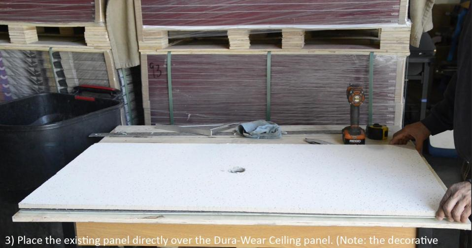
3) Place the existing panel directly over the Dura-Wear Ceiling panel. (Note: the decorative side should be facing up.)
