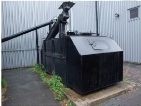
Figure 16, Automatic ash extraction auger from stepped grate boiler and external ash bin
