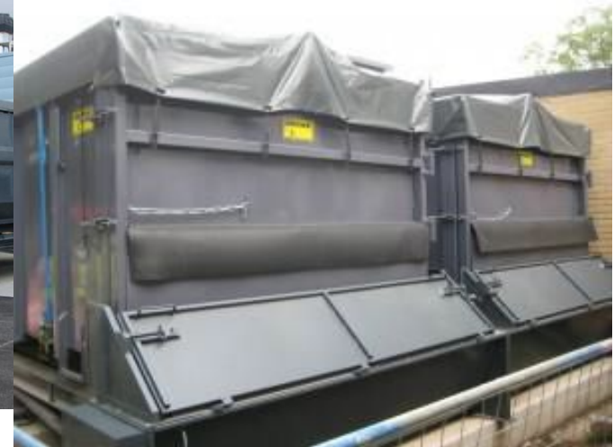
Wood chip hook bins and transverse auger
