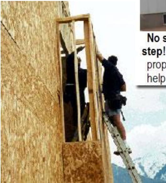
This one seems properly inclined and secured
