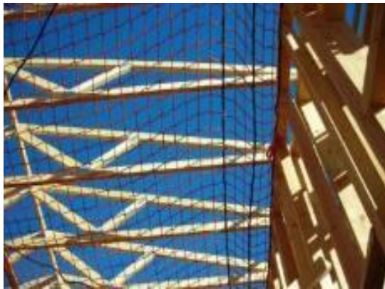
Safety Net in Residential Construction
