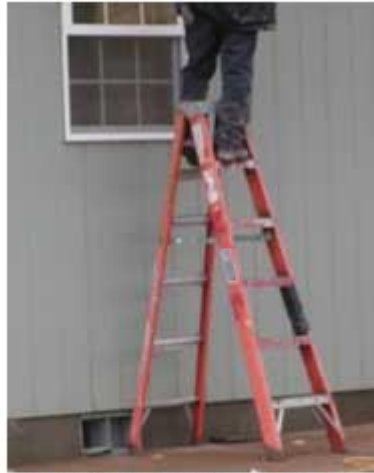
No standing on the top step! Employee training on proper use of ladders will help prevent unsafe use.
