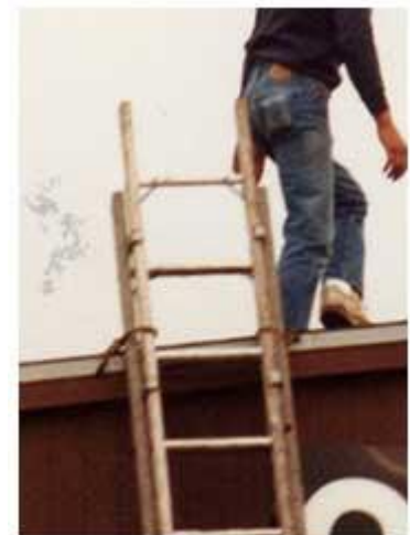
Ladder secured to roof.
