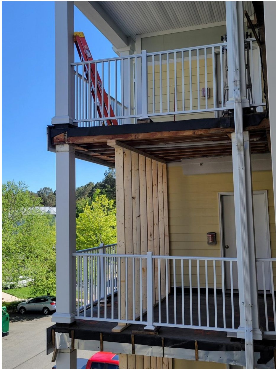
Figure 2 Bracing on second level
