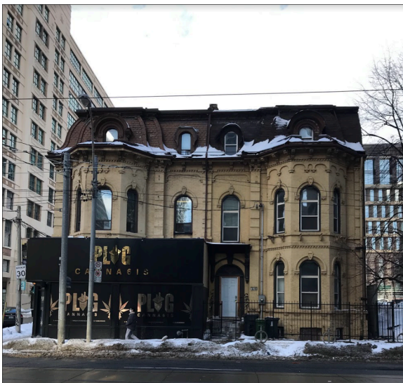
Figure-13: Existing Building on site
