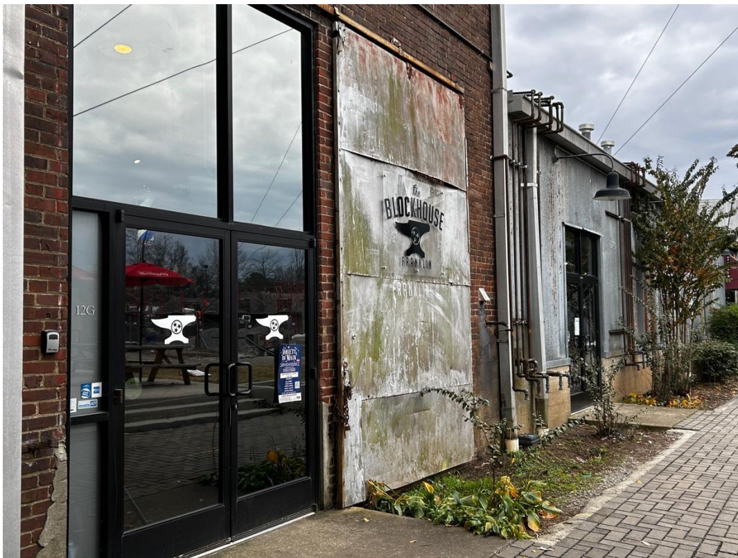
Figure 7. Large industrial door incorporated with modern business advertising and building elements; Shelby Walker, personal photo, November 30, 2024.
