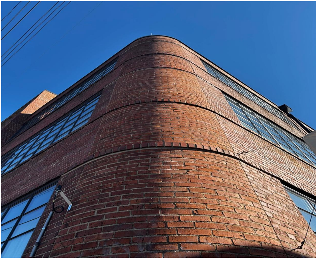
Figure 5. Curved Brick Corners of Primary May Hosiery Mills Building ; Shelby Walker, personal photo, December 5, 2024.
