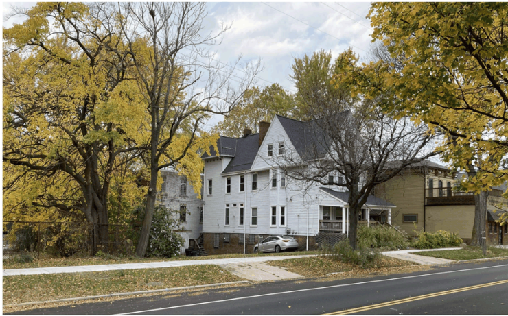
Context Photo View of site and adjacent properties looking NE on Franklin Blvd
