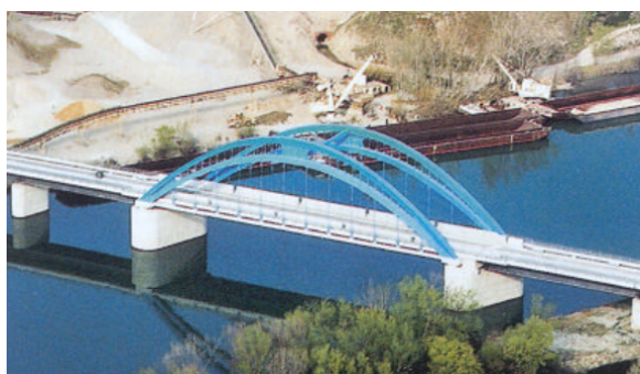
Fig. 3. Multiple arch bridge, where external arches are connected to internal arches through hangers.
