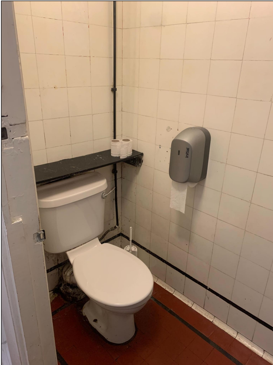
Close up of stall inside toilet with urinals
