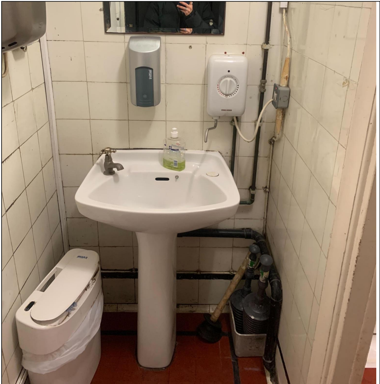
Sink inside stall of toilet with urinals and stall
