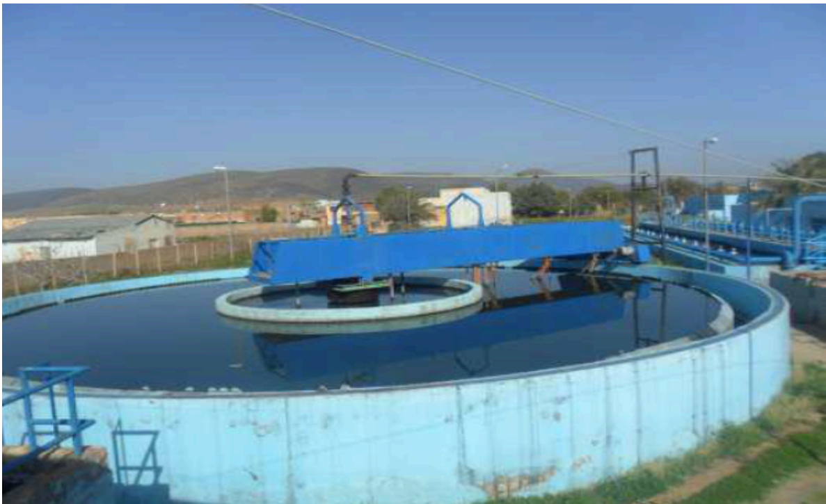
Figure 4. Clarifying flocculator.
