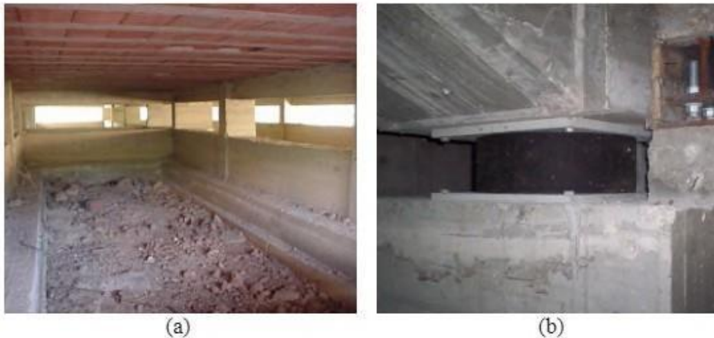
Figure 19: Squat columns in the original building before (a) and after (b) the insertion of the seismic isolators (After Calio and Marletta [28]).
