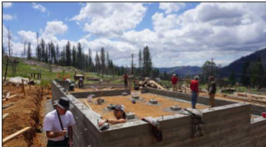
A home being rebuilt as part of the Hope City project in Lake County. Photo Credit: Lake County News
