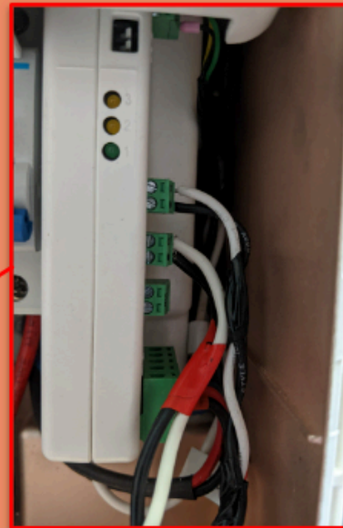
CTs around BUI feeder conductors Arrows pointed back towards feeder breaker
