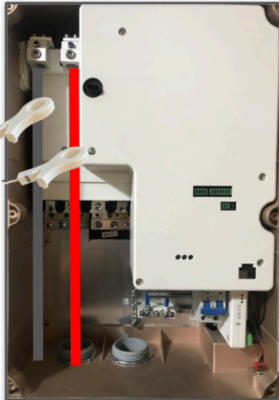
Backup PCS: BUI meter measures BUI feeder
