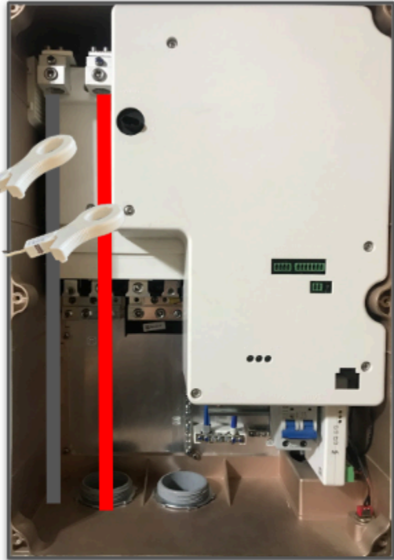
Backup PCS: BUI meter measures BUI feeder
