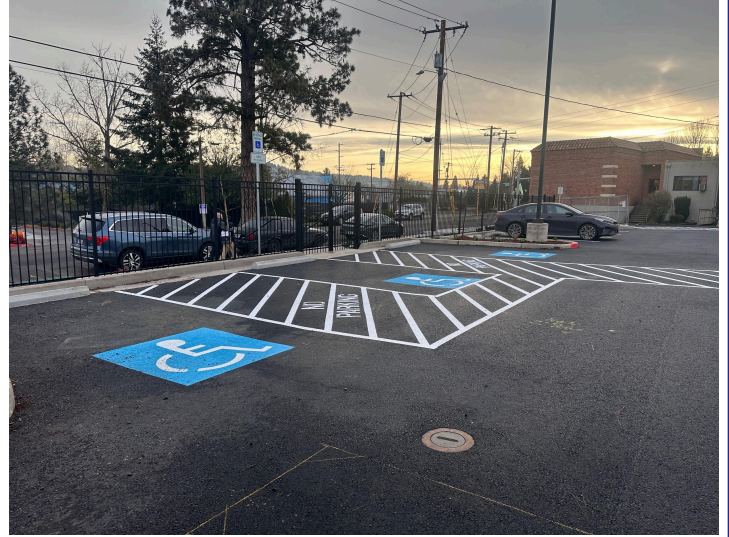
Initial Parking lot striping completed!
