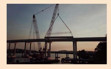
The bridge has a total length of 888 meters (2,913 ft), consisting of seven steel truss spans of 43.1 meters (141 ft) length and twenty-seven steel girder approach spans. The deck carries two lanes of traffic and a footway. One of the steel truss spans is a vertical-lift span, which allows vessels to navigate the Clarence River. However, this now occurs infrequently.
