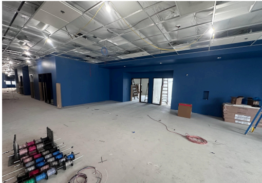
Flex Space on 2nd Floor...Ceiling grids going in...
