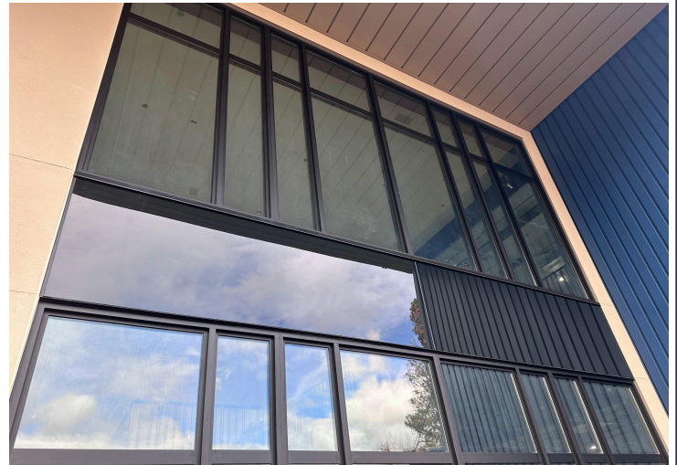
Spandrel glass put up between the windows for a clean professional look
