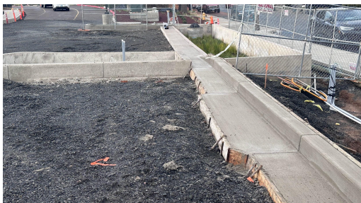
New sidewalks going in...due to the rain, the concrete pour was pushed back to next week.
