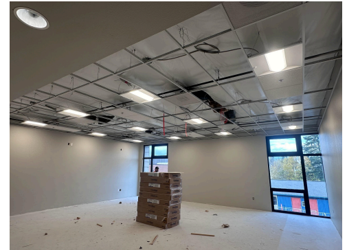
Lights and ceiling grids in classrooms. Next up...the ceiling tiles
