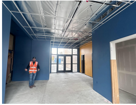
Vestibule between middle school and new building
