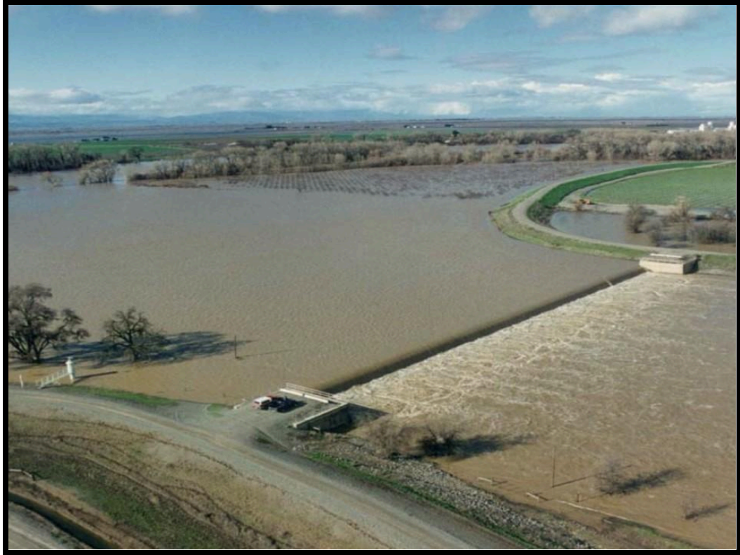
Figure E-4. Spill over of the Moulton Weir from the Sacramento River into the Sutter Bypass in winter, 1997. Adult sturgeon enter (are attracted to) the lower exit of the bypass and are then blocked by the weir as they attempt to return to the Sacramento River.
