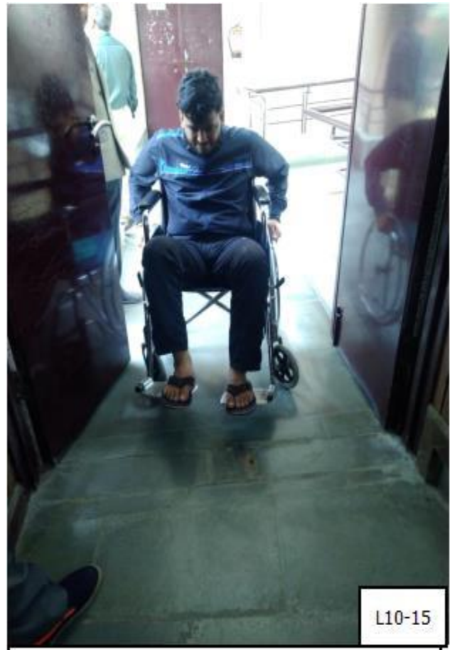
Enough space at door and in front for wheelchair
