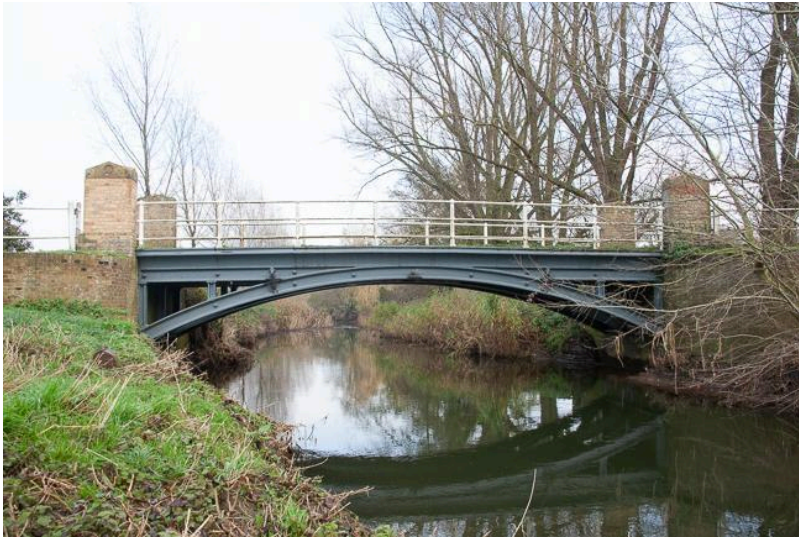
Wormingford bridge, over the River Stour, built 1891 (photo taken in 2020)
