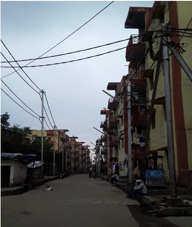
Housing provided to residents of Gautam Nagar
