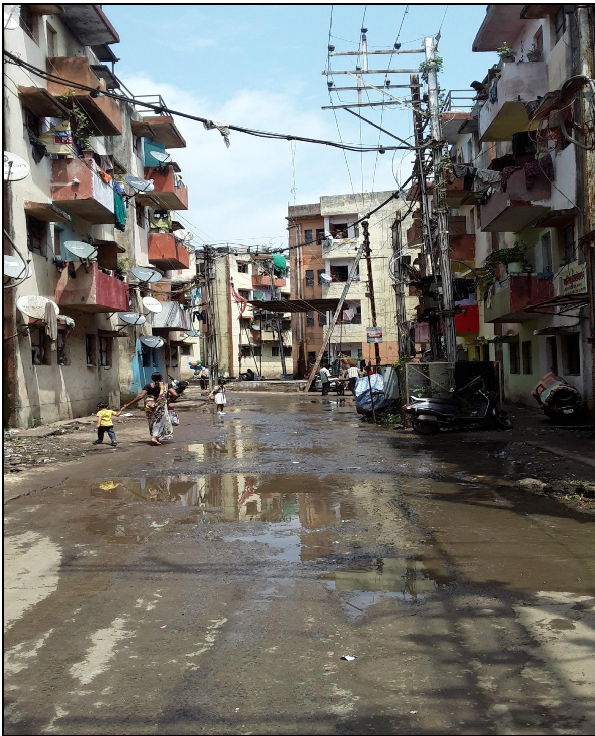
Water overflowing from water tanks
