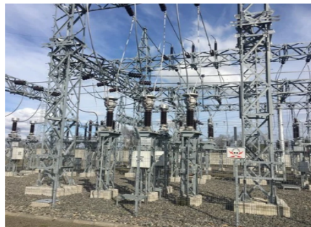
Lattice Steel Structure
