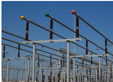
Tubular Steel Structure
