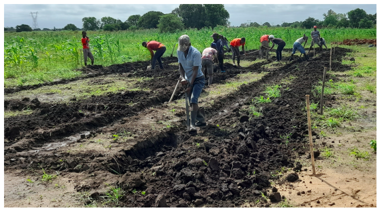
Prepping for the foundation to be laid was a community effort!
