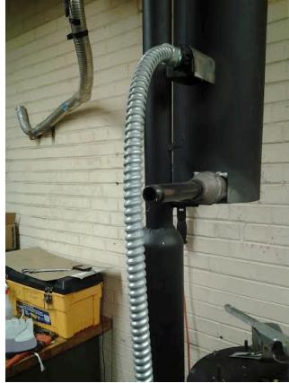
fig1. venturi connections were opened and cleaned
