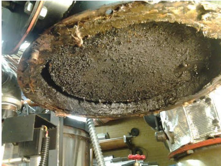
Figure 7. Bottom of the Fuel Hopper
