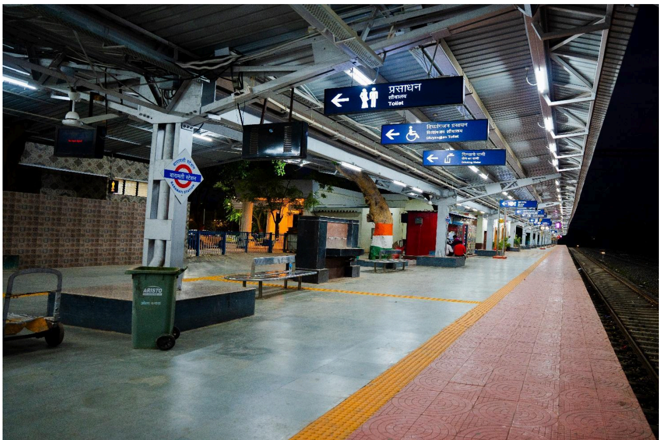
Platform Surfacing and Cover Over Platform
