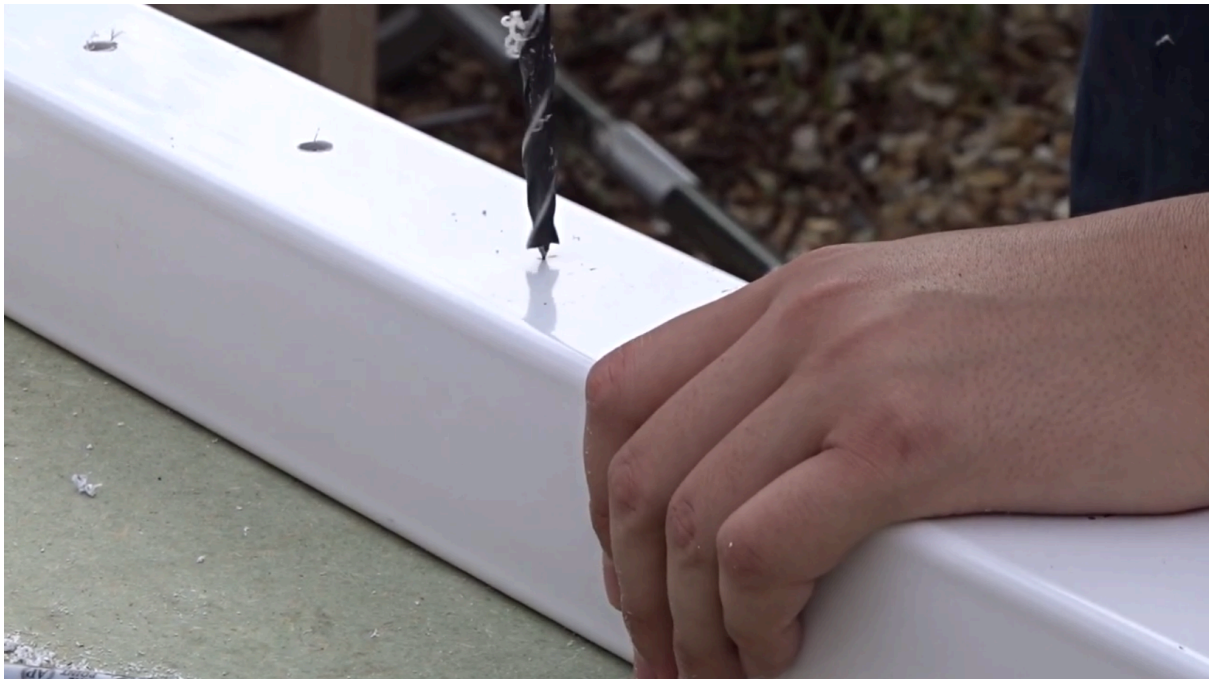
5. Pre-drill with 8mm drill bit.
