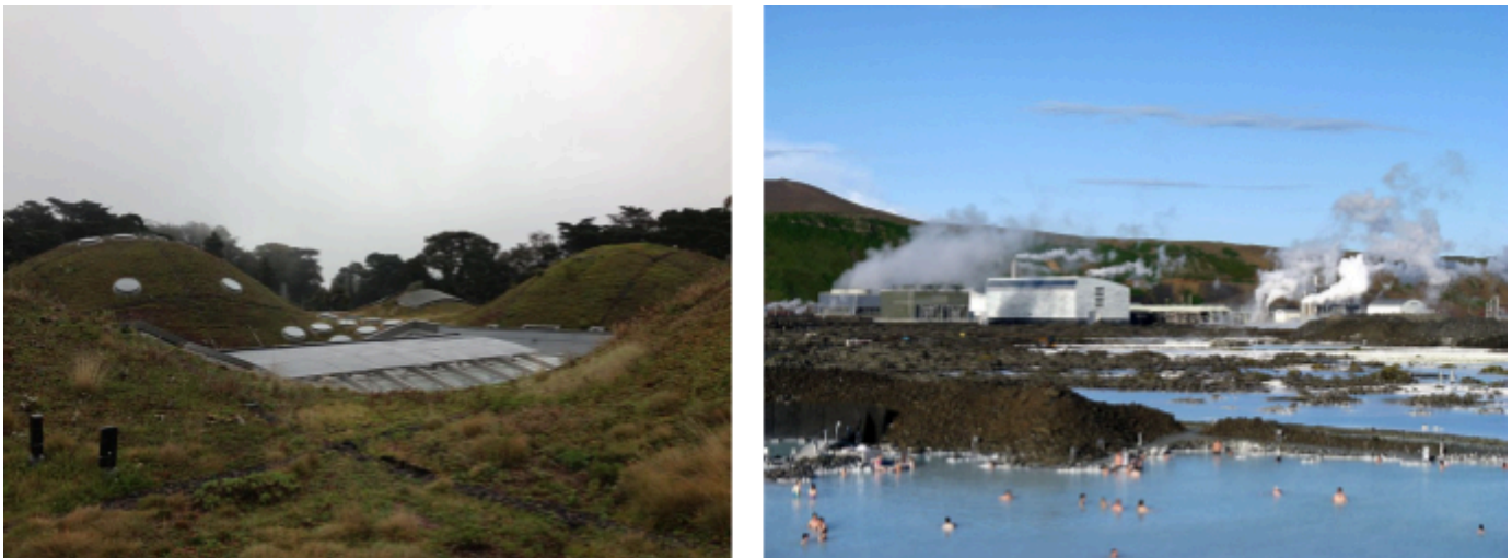
Figure 4 There are a wide variety of electricity solutions. On the left is the living roof of California Academy of Sciences in Golden Gate Park. It provides insulation for the museum below. On the right is a geothermal plant in Iceland. Geothermal power plants produce 25% of that country's energy.
