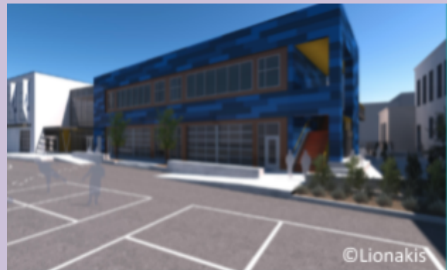
Figure 5 What does a ZNE building look like? Take a look at SFUSD's first Zero Net Energy building at Claire Lilienthal School on Divisadero St. It will generate all of the energy it uses on site!
