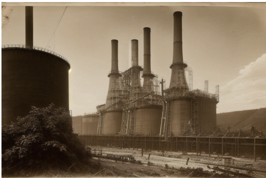
picture 2: coal power plant under construction in Kaal Naareyen, 1893, old photo
