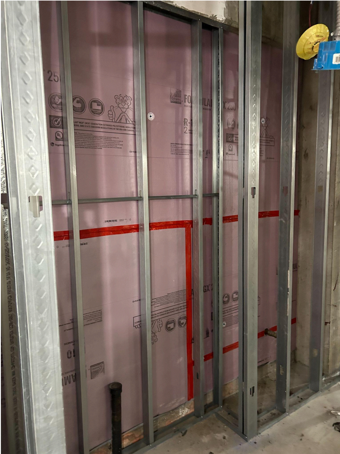
Insulation installed on the interior of the exterior walls over the old block walls that framed the exterior walls for the 1965 wing of the building.
