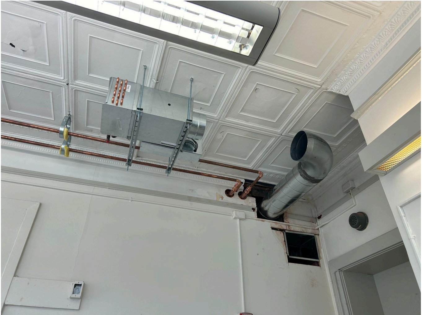
Another picture of the ventilation equipment and ductwork being installed in the classrooms of the 1904 wing of the building.
