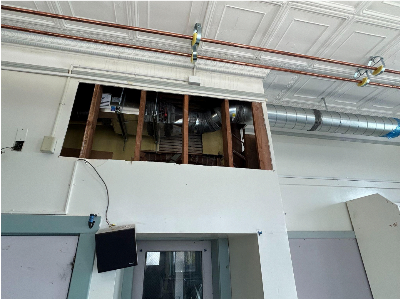
VMI is installing the ventilation equipment and ductwork in the classrooms of the 1904 wing of the building.
