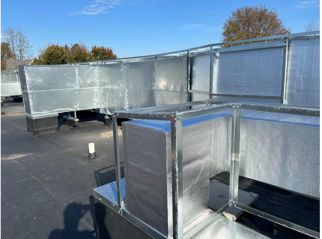
A picture of the ductwork that has been installed on the roof of the 1965 wing of the building that is being covered with sheetmetal to protect the ductwork and insulation. The shiny sheetmetal will be painted in the spring.
