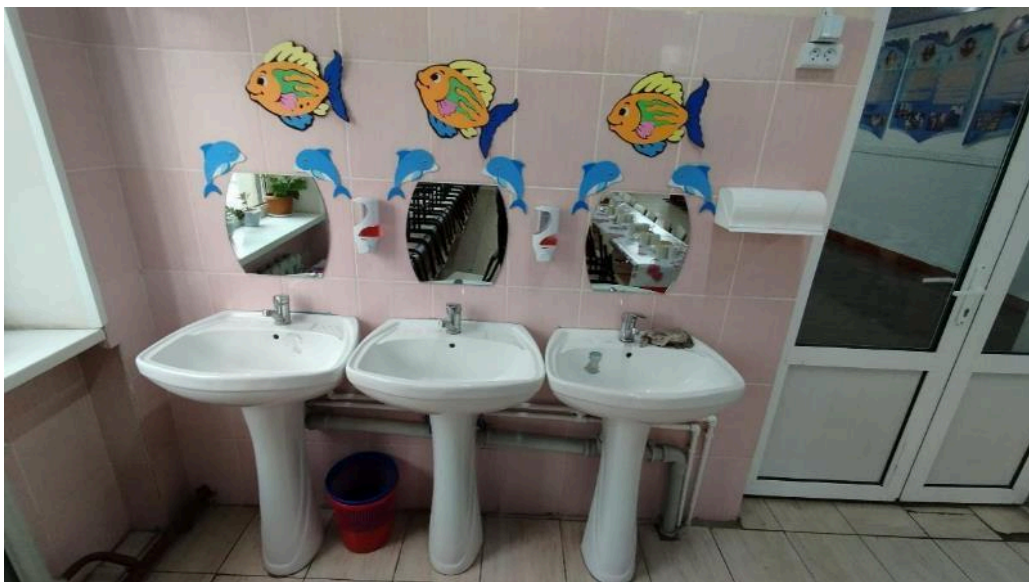
Photo 6. Washbasins in the canteen
