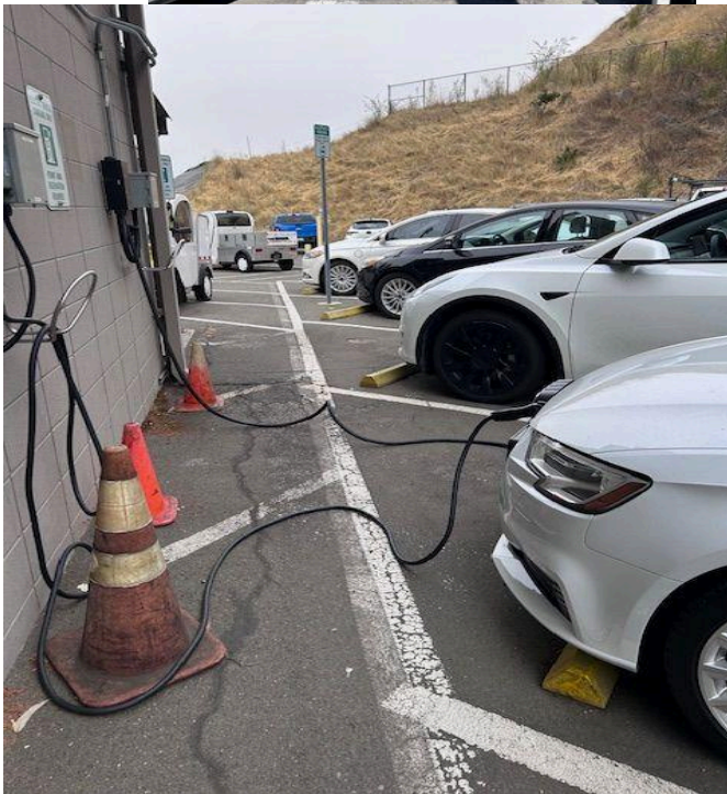
Cord looping in walkway - Incorrect Corrected Cord Management
