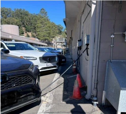
Incorrect cord draping across walkway
