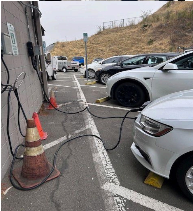
Cord looping in walkway - Incorrect
