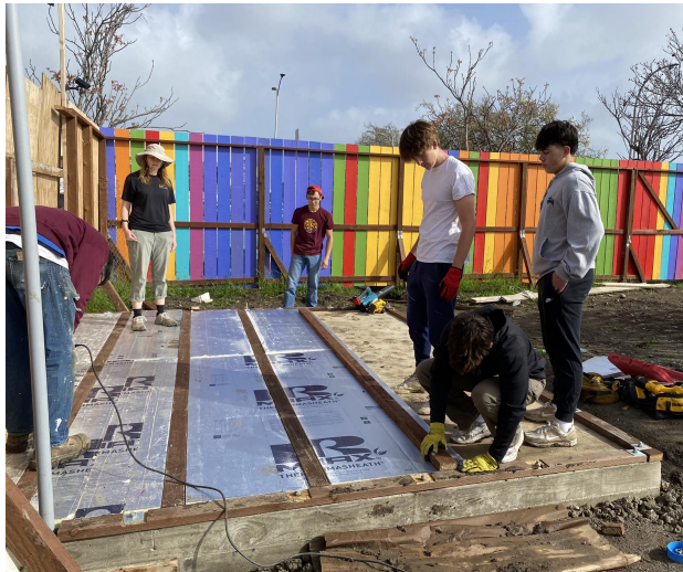
Photos: Feb 2025: welcome center foundation
