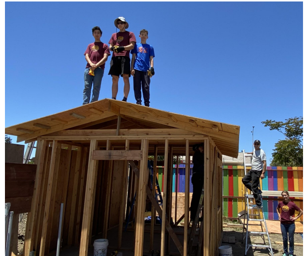
July 2025: roof in place
