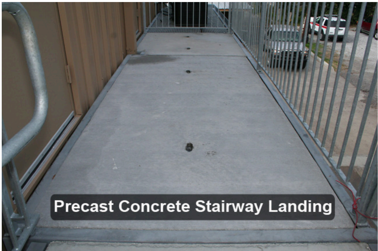
Figure 10: Landings at the top and bottom
