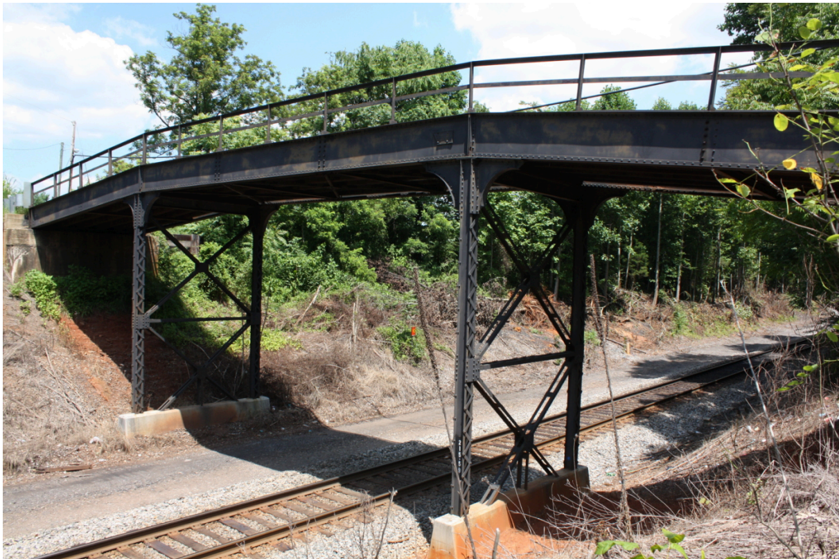
Figure 17: There is an overpass above the tracks
