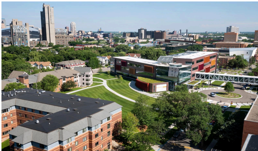
An aerial view of the western edge of Augsburg University's campus, with the Hagfors Center For Science, Business and Religion seen center-right and the Courtyard Marriott above it.
