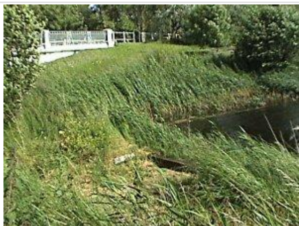
Wharf at Mights Bridge
