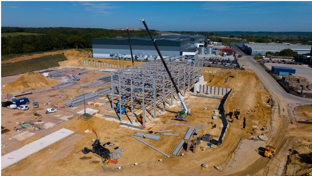
The steels are now in the ground at the Suffolk Port One Logistics Park for the Hemisphere Freight Services Build
