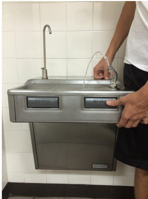
Rec - Room 125 Temp=11 C Stream=5 Height=2 Quality=4 Bottle Filling=4.5
