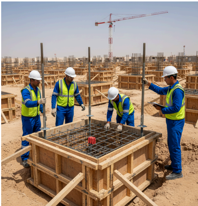
INFORCEMENT STEEL & CONCRETE WORKS
