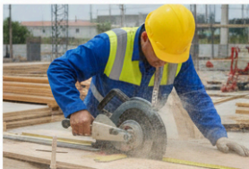
1. Preparing Plywood Panels
