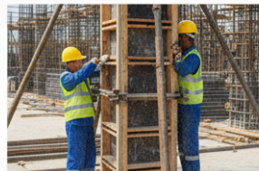
2. Erecting of Bracing Column Forms
