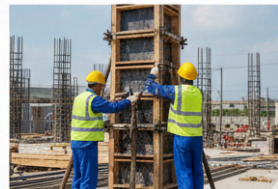
2. Erecting of Bracing Column Forms
