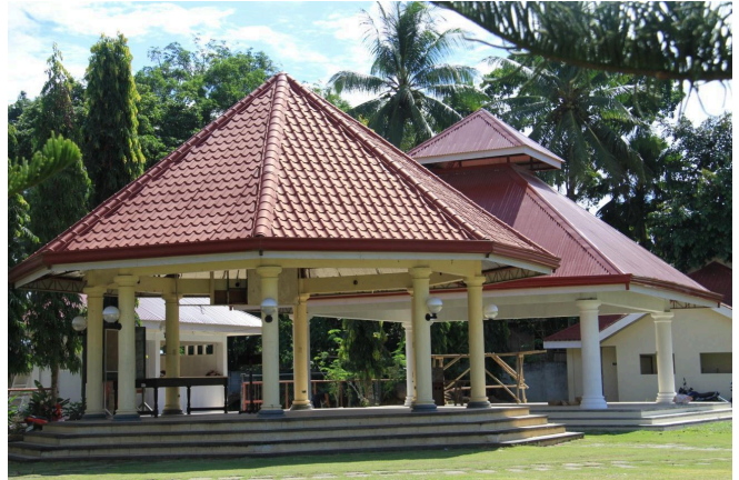
The two gazebos with the toilet/ dressing room visible at the far side
