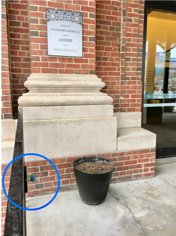
Image Description: Very small, round blue automatic door button mounted on a black metal railing to the left of the Miller High Life Theater's main entrance. A blue circle has been added to the image to highlight the automatic door button.
