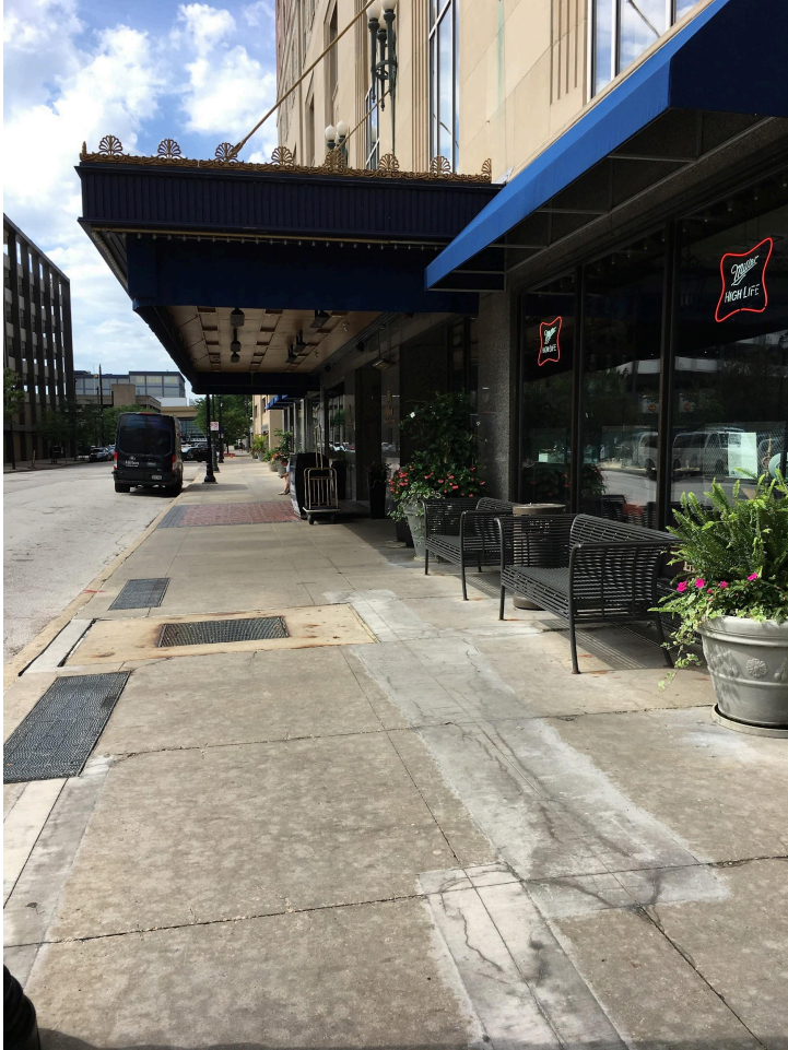
Image Description: Exterior of the Hilton's 5th Street entrance. There is a curb with no curb cut between the sidewalk and the street, and a large flat awning.
