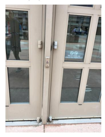
Image Description: A small automatic door button for the far right door of the Wisconsin Center main entrance. The door button is located on the door jamb just to the left of the automatic door.
