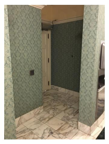
Image Description: Tight entryway to Hilton 4th floor restroom, requiring two 90 degree turns in a 30-inch pathway. The tile is white and gray marble, and the walls have a sage green brocade pattern.
