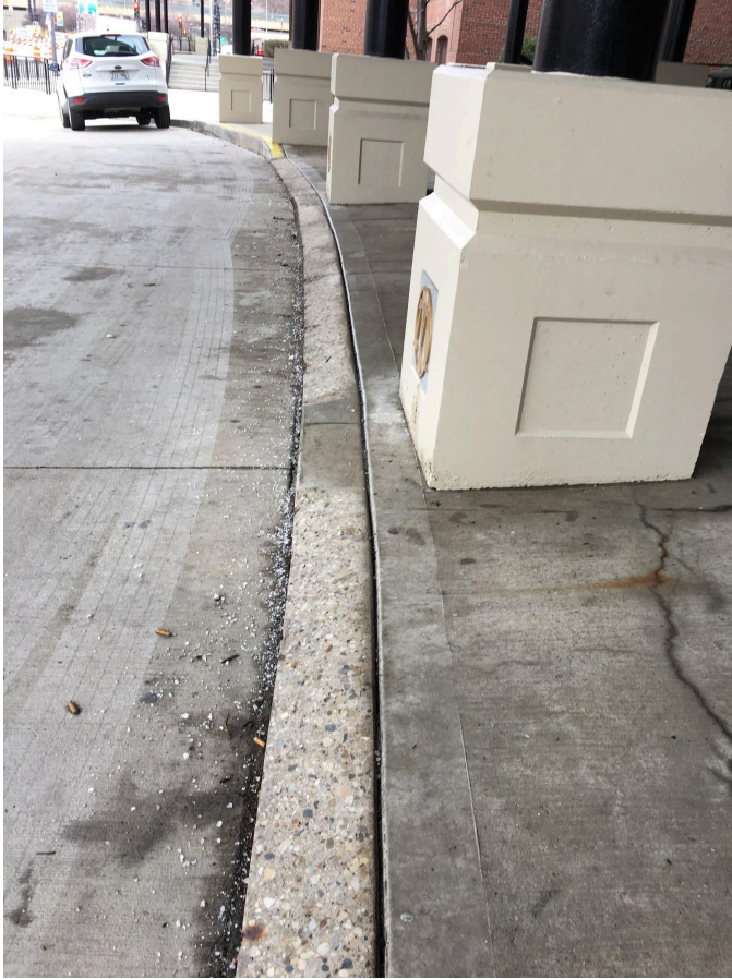
Image Description: Rough-hewn curb cut between the driveway and sidewalk at the Miller High Life Theater entrance.
