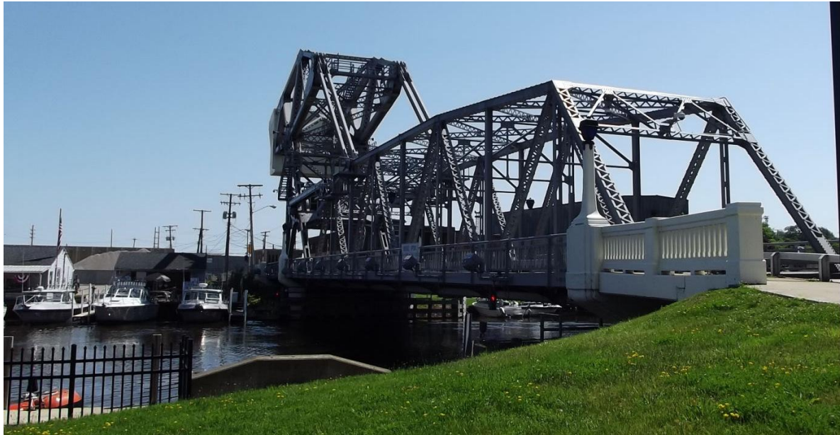
Ashtabula lift bridge, photo taken by Jack Schmidt in June 2015 for Bridgehunter.com
