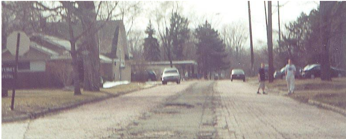
Old US 20 with its bricks and asphalt center, west of Geneva. March 21, 2001 photo from Roadfan.com
