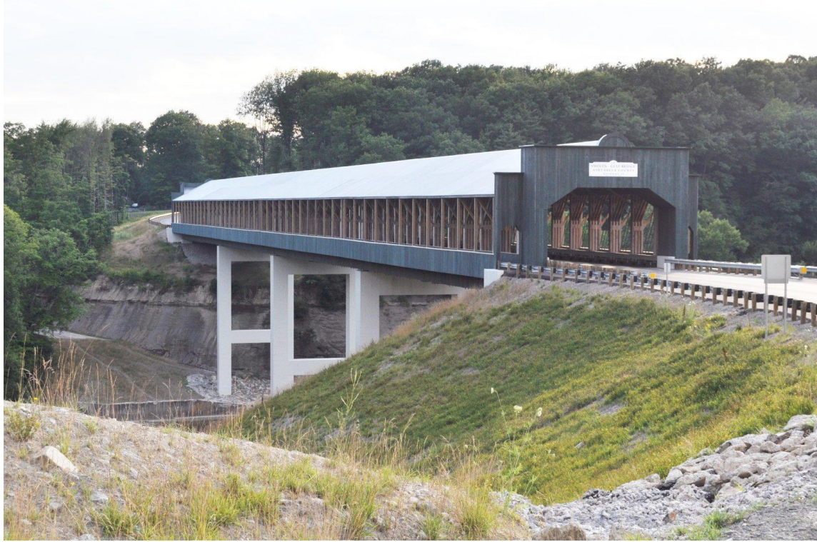
Smolen-Gulf Bridge, July 2009 photo by James Baughn for Bridgehunter.com
