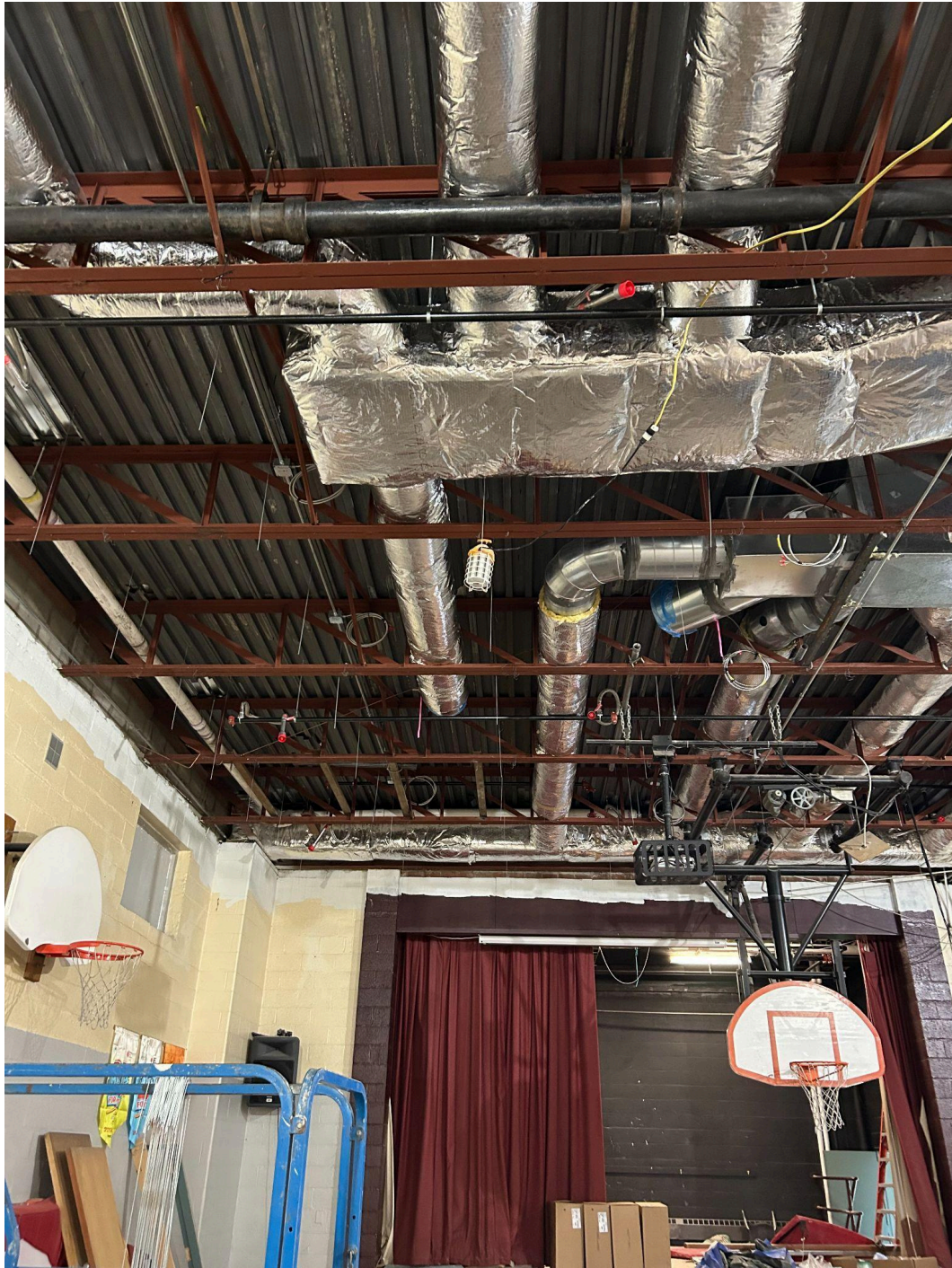
Wires stub down from the ceiling of the GYM to accept the installation of the new ceiling grid that will be installed.
