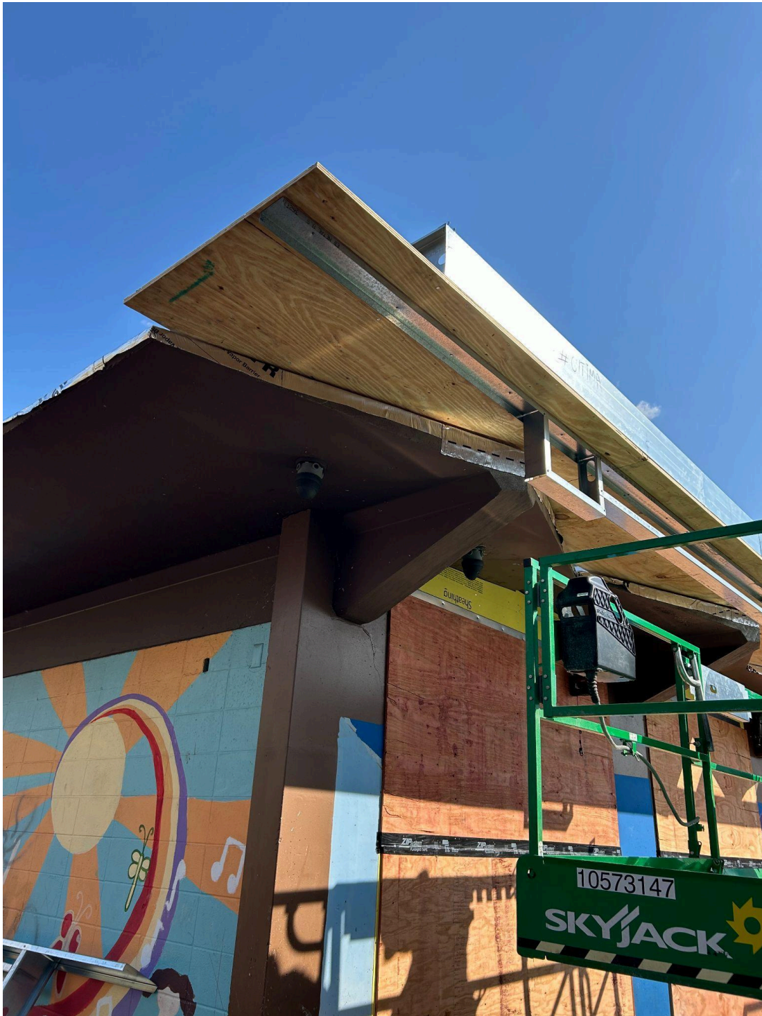
Optimum Construction has started the underside or soffit construction at the back corner of the 1965 wing of the building.
