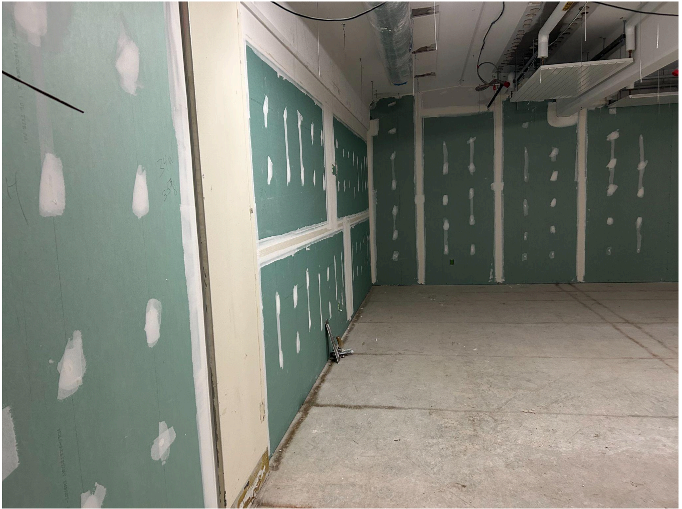
The Finish Contractor has started the first coat of mud on the sheetrock seams of the classroom walls that are on the North end of the 1965 wing of the building.
