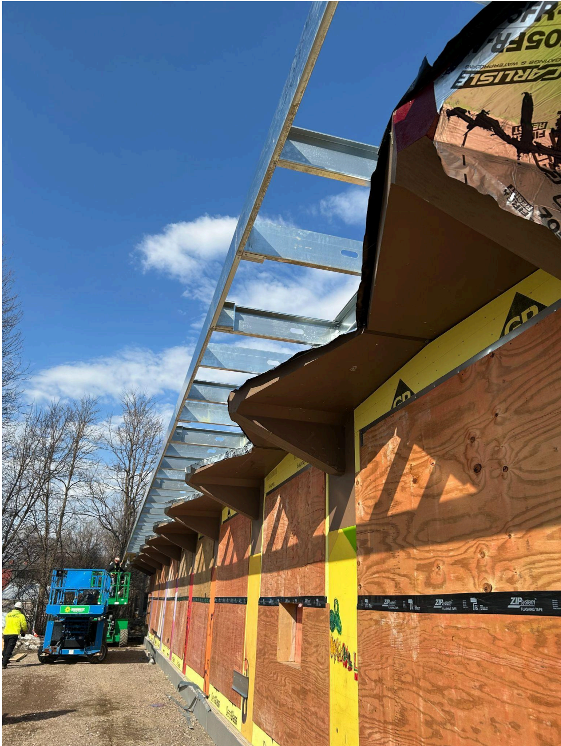
A picture of the “squaring off” on the underside of the roof framing.
