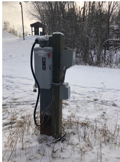
Outlet at near stand pipe.
