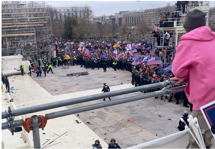
Same time, before full breach, shot from NW scaffolding (note that the South scaffolding has no white covering, while the North scaffolding does)
