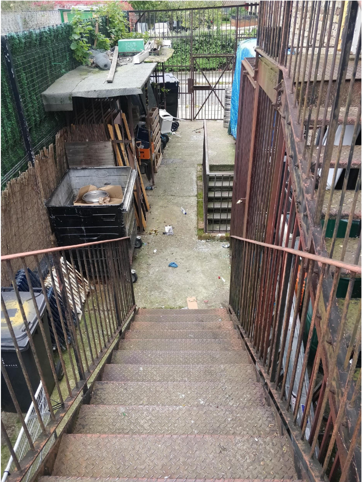
Image description: Metal fire escape steps into bin area and then onto street
