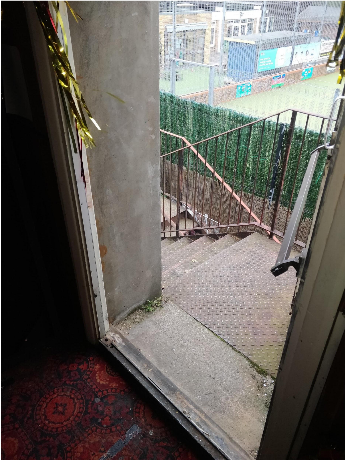
Image description: Fire exit doorway from performance space, with step over onto metal fire escape stairs
