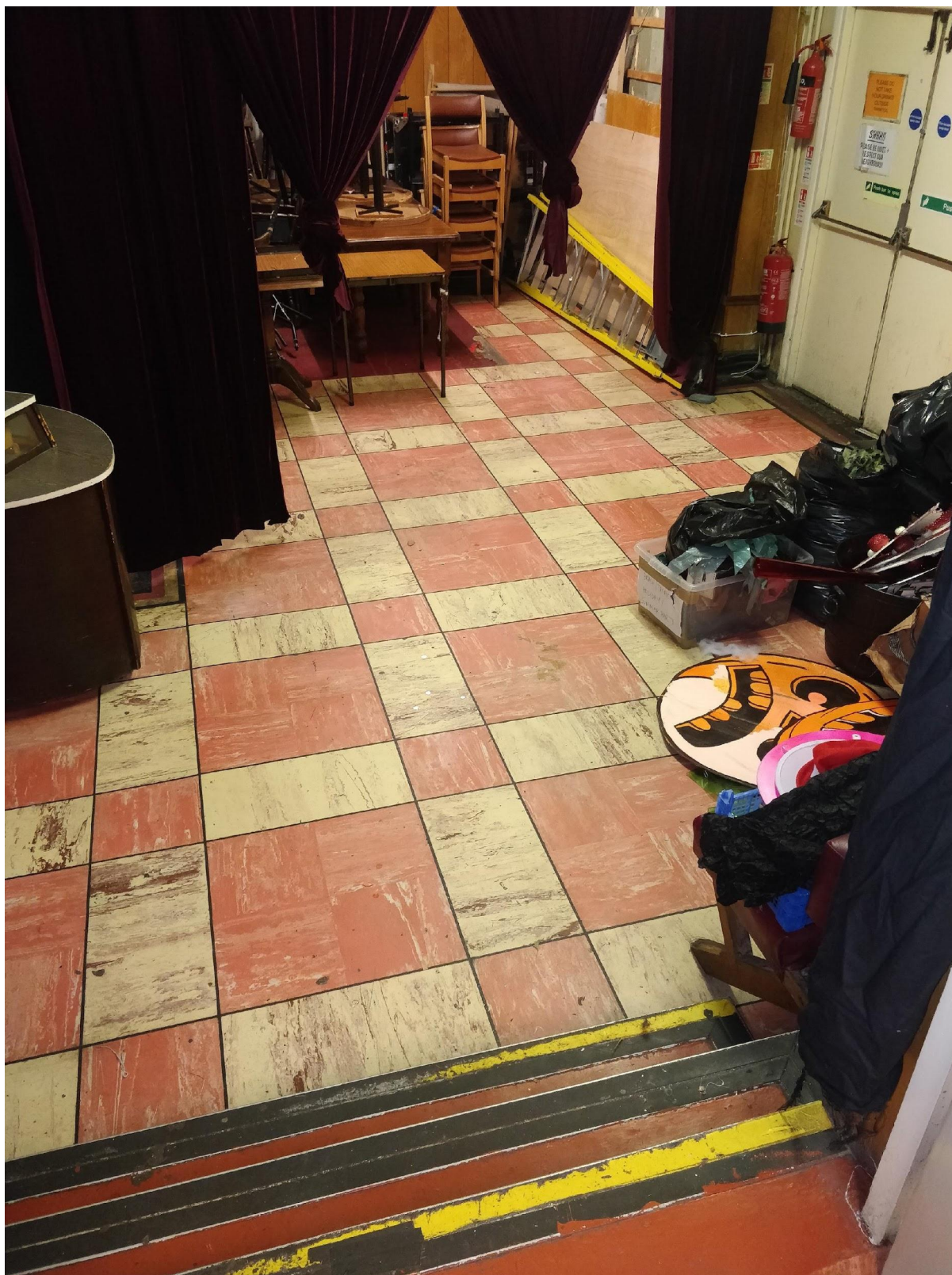
Image description: 3 steps from lower level down to access smoking area (through double fire doors)
