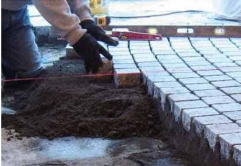
Fig. 4: Setting Bed for Installation of Bricks
