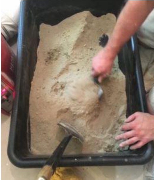
Fig.: Dry Pack Mortar before adding Water
