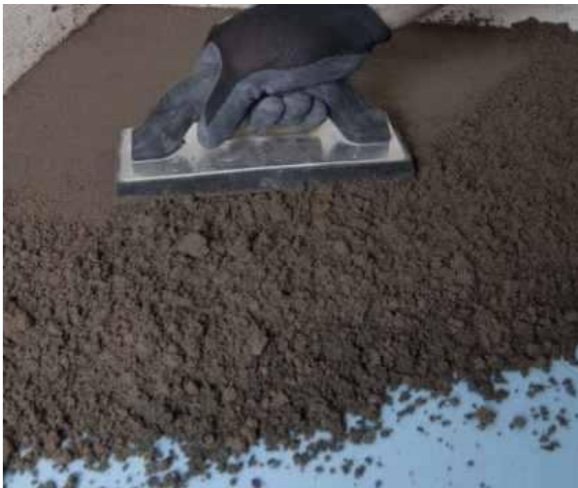
Fig. 5: Creating Bed for Shower installation
