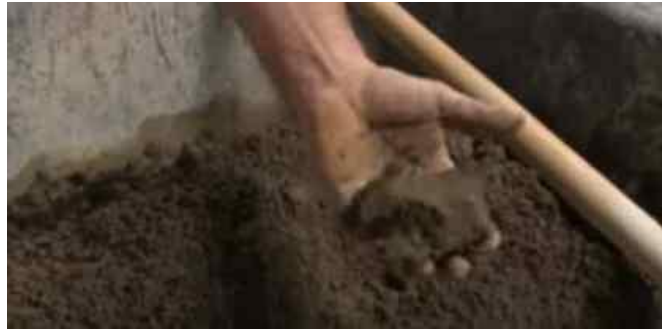
Fig.: Adequate amount of Water added
