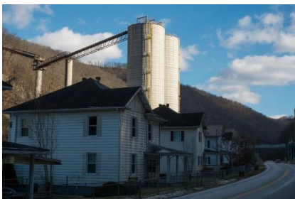
Coal silos behind coal camp houses in Stirrat, West Virginia. The mine is owned by Alpha Natural Resources, which purchased Massey Energy in 2011. Roger May for Al Jazeera America
