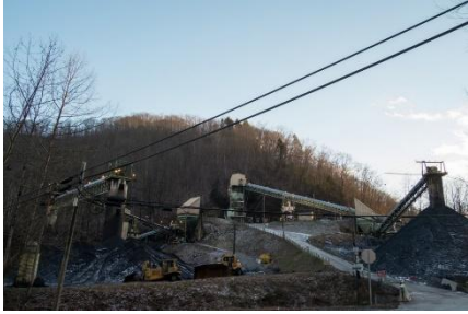
Blackhawk Mining Mingo 2 Loadout facility near Gilbert, West Virginia. Roger May for Al Jazeera America
