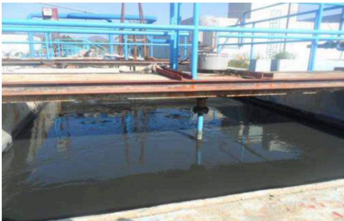
**Figure 3.** Mixing and neutralization basin N ° 2.
