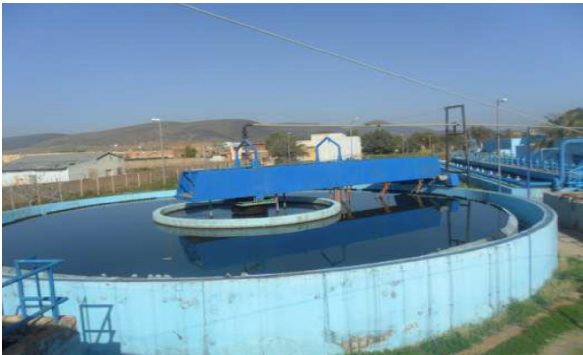
Figure 4. Clarifying flocculator.
