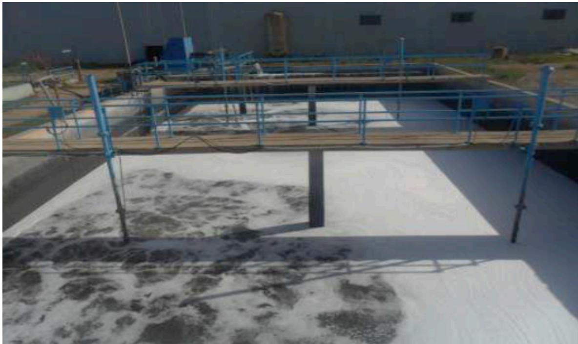
**Figure 2.** Photo of mixing and equalization basin N ° 1.
