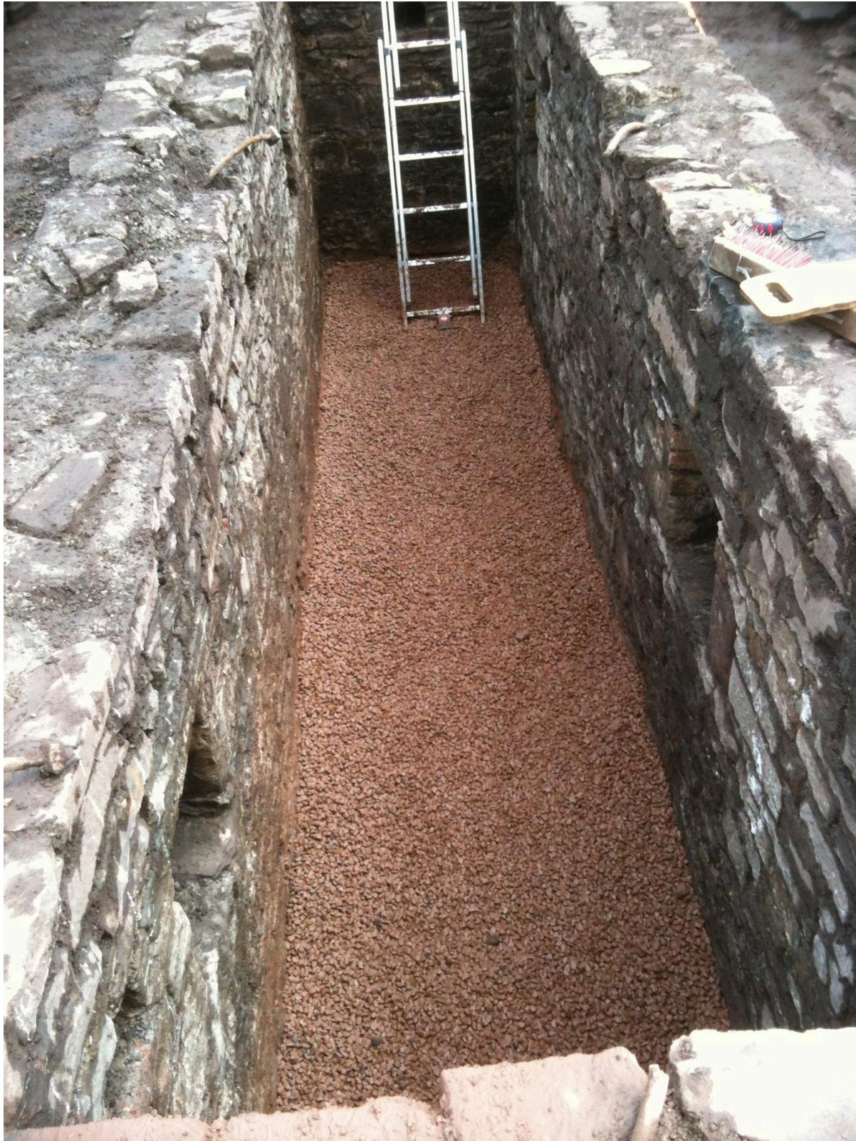
Pit area all cleaned up now , we think it was used for sawing 5 meter long tree trunks into logs for making lock gates.
