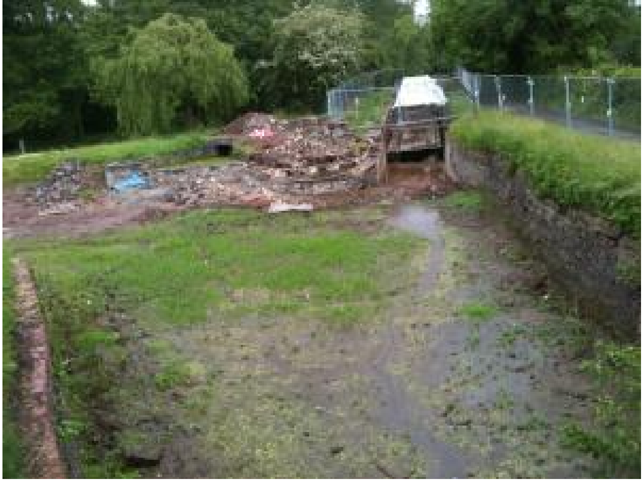
A view of the work being done by the canal restoration team on one of the locks
