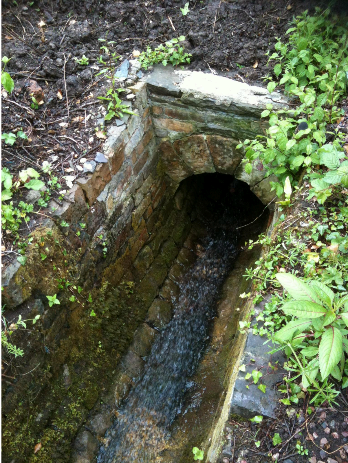
It flowed into a very well preserved culvert
