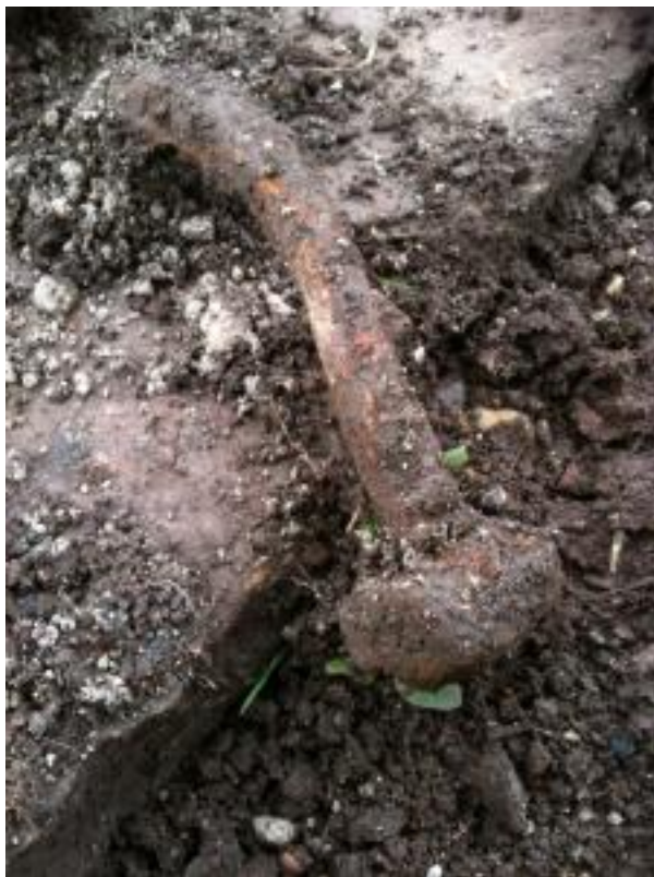
One of the large iron bolts and hand made nuts , but what were they for? We have found several of these embedded in the foundations
