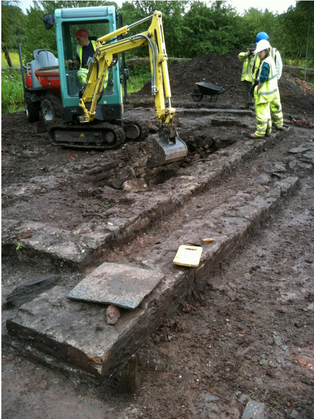
11 am . Excavation of the hole was done by machine – far too much work to do with hand tools
